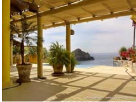
Washed cement floor and pergolas
