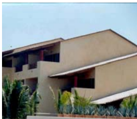
Inclined coverings with tile roof
